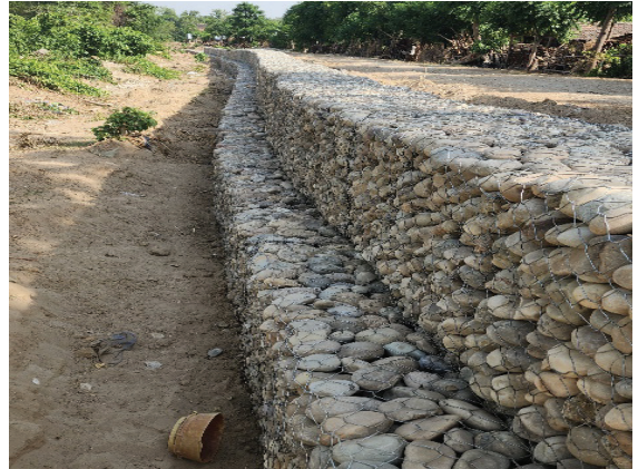
Figure 12 Check dam Installation-Jalandhara CFUG-Dhakeri, Banke
