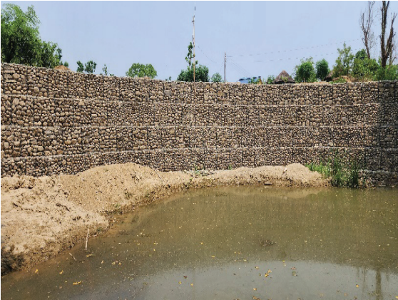
Figure 11 Check dam Installation-Sadabaha CFUG-Mehemenpur, Banke
